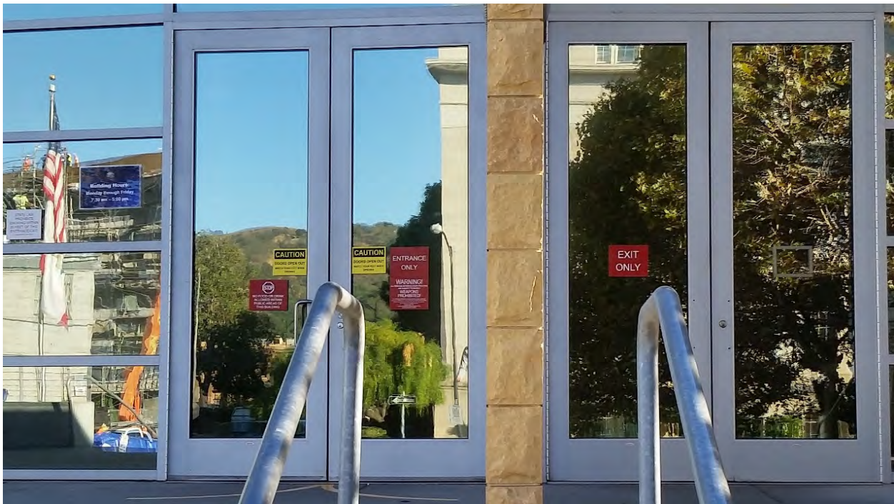
Figure 9. Entrance to the Spinetta Family Law Center, showing affixed signs regarding building hours (created by court manager), and entrance and exit signs (in red) with brief weapons warning. There are two other signs (in yellow) indicating doors open outwardly, and a white sign with text regarding non-smoking law.
